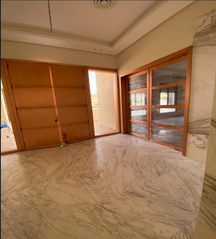
Marble and joinery finishes
