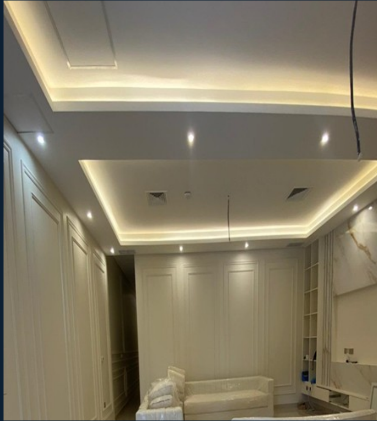
Decorative ceiling and wall details
